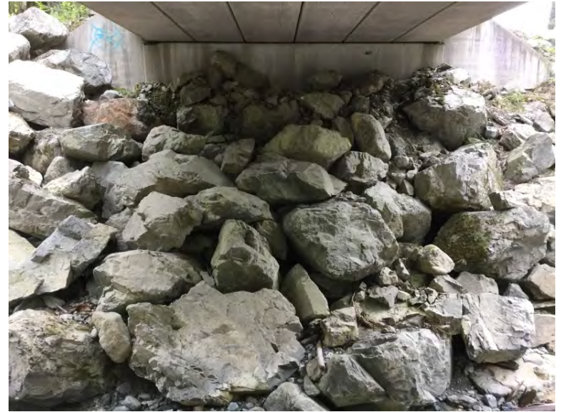
Left Bank Abutment when facing downstream
