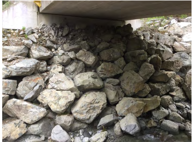
Right Bank Abutment when facing downstream
